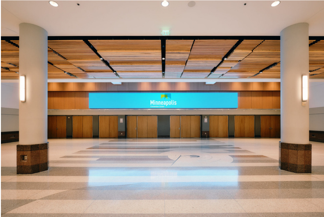
View from middle of Lobby looking towards doors to Auditorium.
